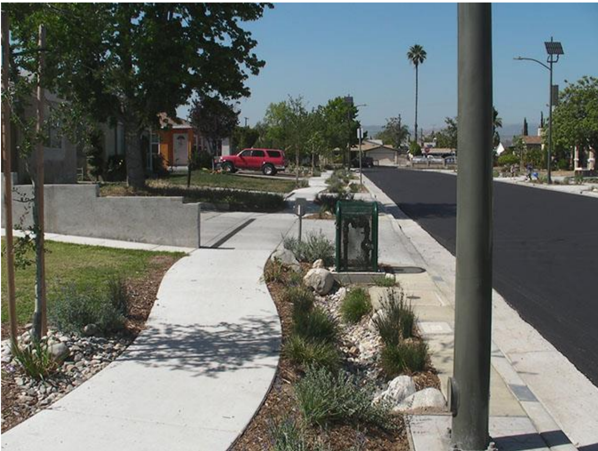
Figure 1-8. Sidewalk and bioswale in the completed public right of way after the Elmer Avenue Neighborhood Retrofit in Los Angeles, California.
