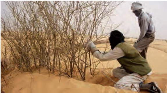
Figure 1-7. Dune stabilization in Mauritania.
