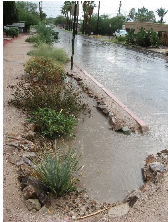
Figure 3-1. A curb cut draws stormwater from the street into a bioretention basin in the right of way.
